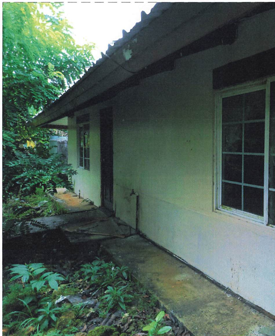
LEFT SIDE VIEW (WATER TANKS AT THE REAR)
